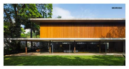
The ground floor of sliding glass walls and 14 slim steel pillars supports an upper floor box of wooden screens that filter the light, so that the house appears to float over the landscape.
